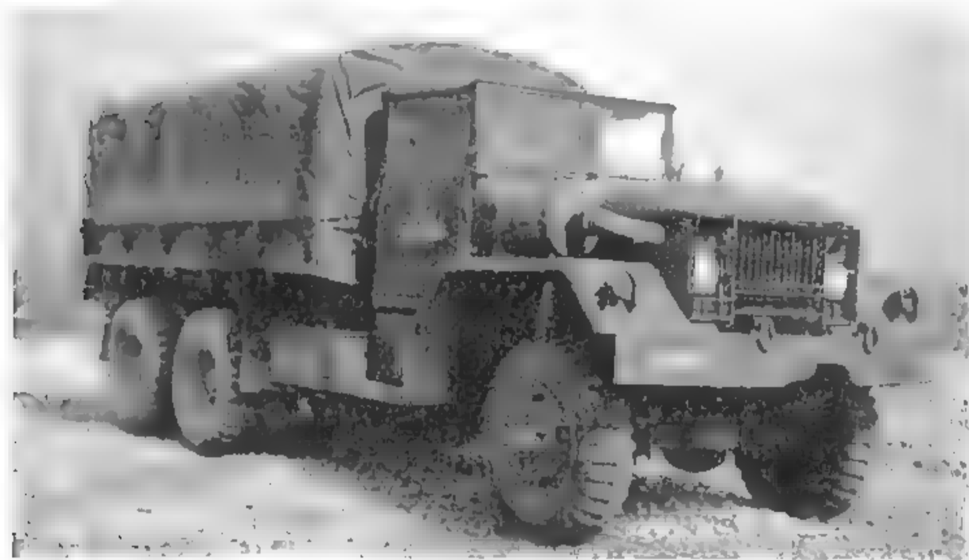
The M54E3 was the test bed for installing the Mack ENDT-673 engine in the 5-ton cargo truck. (Photo courtesy of the Patton Museum).
